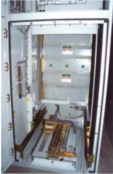
Arc-Resistant Circuit Breaker Compartment
